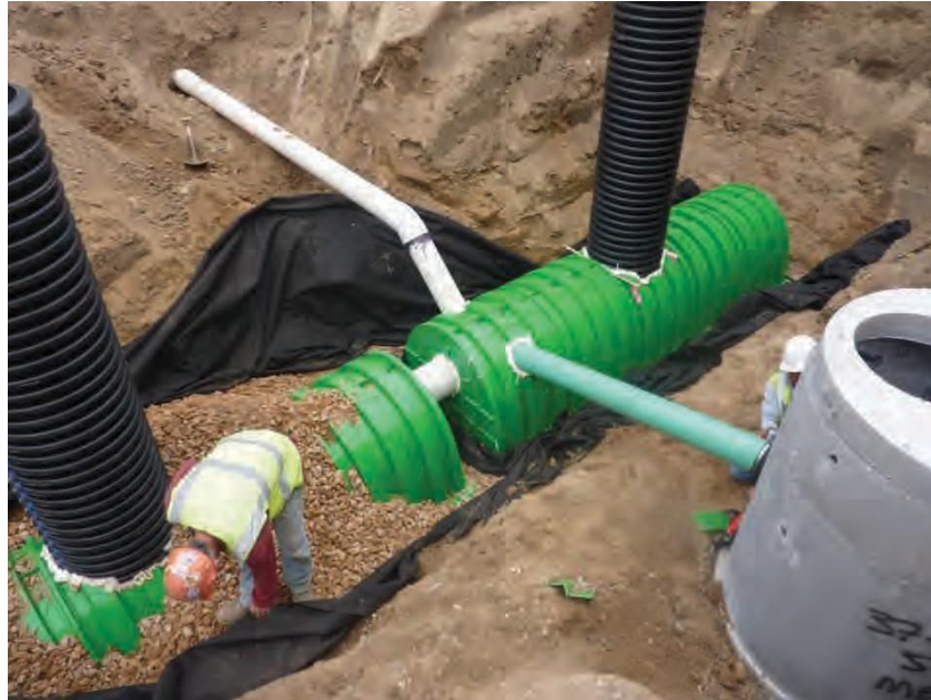
Figure 4 - Triton Header Row with direct chamber connection for maintenance and inspection (Top Access), end connection and inlet top/side connections.
