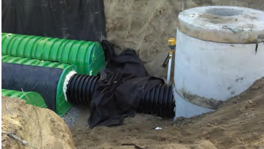
Figure 5 - Triton Header Row with manhole connection for maintenance and inspection (End Access)
