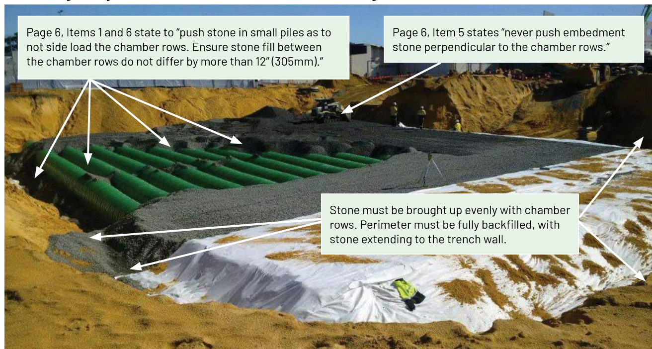
Non-recommended backfilling of system.
