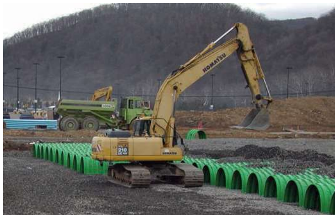
Installing embedment stone around chambers.
