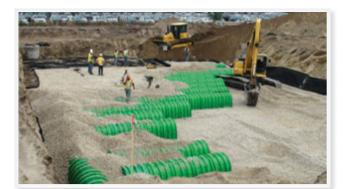
The site of the water retention system is backfilled up to six inches past the crown of the chambers.
