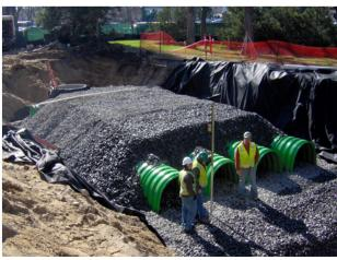
Both site locations utilized a single-tier chamber design with Main Header Row. Typical of most installations, geofabric was used to line the sides of the trench and crushed stone was used to backfill around the chambers. In total, more than 41,000 cubic feet of storage was produced with a footprint of just over 10,000 square feet.
