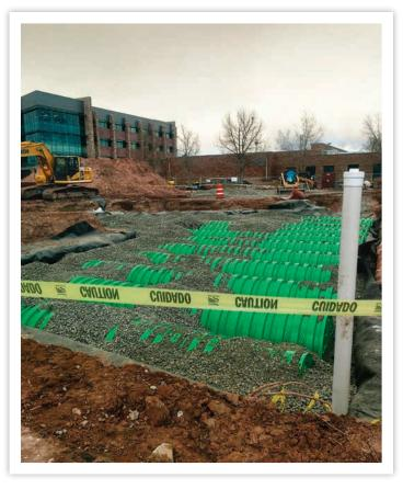
The stormwater management portion of the project was completed in less than two weeks — minimizing hassle to the campus community while creating over 6,000 cubic feet of stormwater storage capacity.
