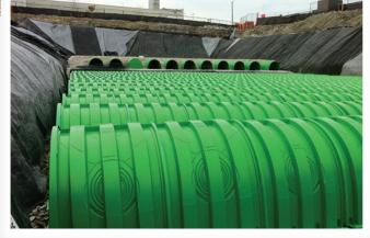
The Triton SWS Chambers lightweight design and ease of installation allowed the project team to place nearly  $2{,}000$  chambers in less than two days.
