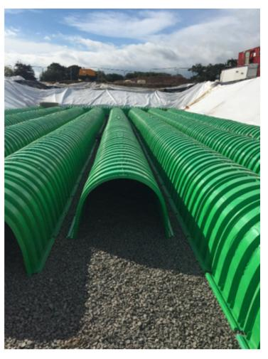
Triton SWS UK Limited were able to provide a system that would be positioned within a central area of public open space. The design utilised two layers of Tritons S-29 chambers which would provide the storage and access requirements for Severn Trent Water.
