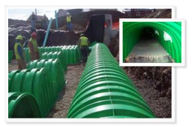
An integral Triton sediment catch basin (inset photo) was built into the Main Header Row.
