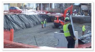
The Dubois project required a storage capacity of 11,500 cu ft of water, in a footprint that is 80' x 50'.
