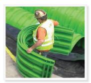
Following the chamber installation, the embedment stone was backfilled to a consistent cover of 6", the finish grade fill was installed, leveled with a backhoe maintaining 8" of cover, and compacted.
