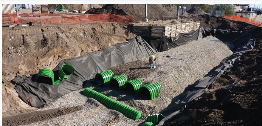
An impressive 10,213 cubic feet of storage was achieved with a 2,837 square foot project site, using Triton SWS’ double-stacking capability.
