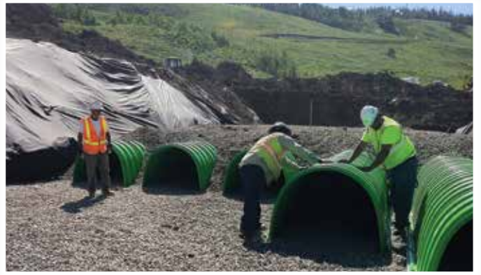
The small installation crew placed chambers to create 35,000 cubic feet of storage capacity in less than a day.
