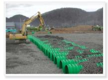
A 15-acre outdoor shopping complex site in Keyser, WV required over 100,000 cubic feet of storage to handle water run off from the parking lot. Triton chambers, which have 46 percent greater capacity, meant fewer chambers were required for the project. This was a key factor in saving costs.
