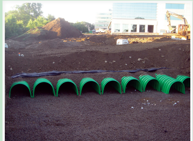
The Triton system supports more weight with less cover.
