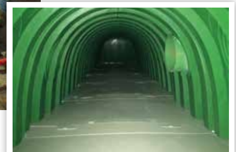
A high voltage duct bank had to be worked around – highlighting the Triton Stormwater Solutions chambers' modular design flexibility. Inset photo shows the main header row floor and interior – an easily maintained sediment removal option.
