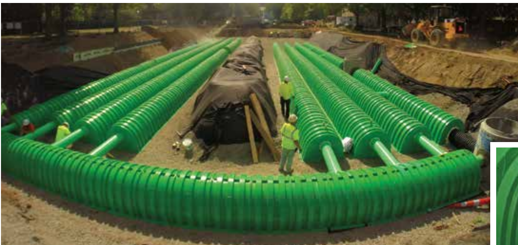
A high voltage duct bank had to be worked around – highlighting the Triton Stormwater Solutions chambers' modular design flexibility. Inset photo shows the main header row floor and interior – an easily maintained sediment removal option.
