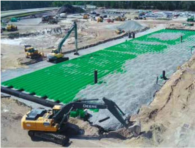
The IKEA project utilized nearly 14,000 Triton chambers, and provided 259,000 cubic feet of stormwater storage.
