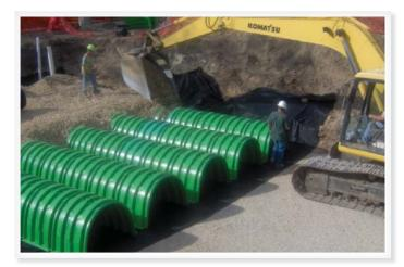
The site is backfilled with stones up to six inches past the crown of the chambers and the geo fabric is folded back down. The Triton system will be under 12 feet of cover after the backfill process is complete.
