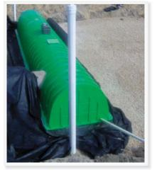
High volume capacity was the driving factor in selecting the Triton stormwater system for the fast food restaurant renovation project. An added benefit of Triton modular design allowed the contractor flexibility to assemble the systems as they had time in between other tasks.
