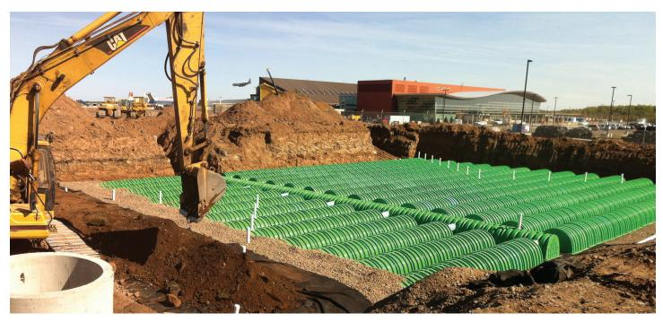
Triton Stormwater Solutions underground stormwater system saved land and helped to eliminate the hazards associated with above-ground retention ponds at Minnesota's Duluth International Airport.
