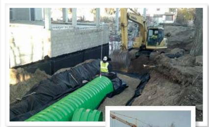
The strength of the Triton system was critical to the project. Developers were able to position the construction crane - weighing over 139,000 pounds with counterweights - over the installed chambers, saving them the trouble and expense of shutting down an adjacent street.
