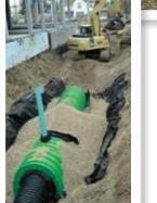
The flexibility of the Triton system allowed developers to create the needed storage with two straight-line systems running along the front and back of the building.
